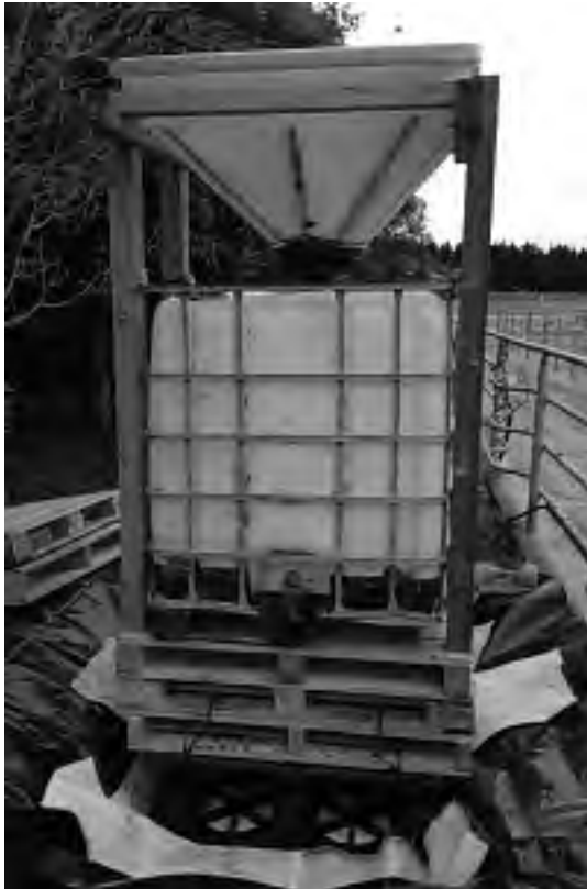
Figure 1: Copper sulfate filter under construction (without submersible pump attached)
